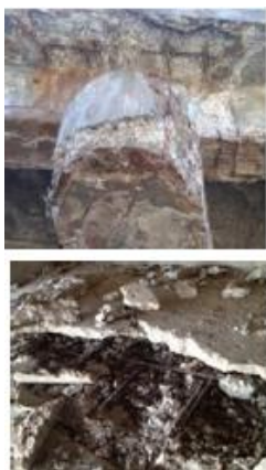
(a) Corrosion of columns
