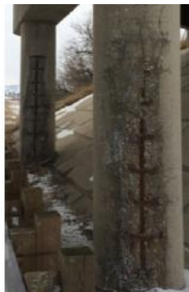
(a) Corrosion of columns
