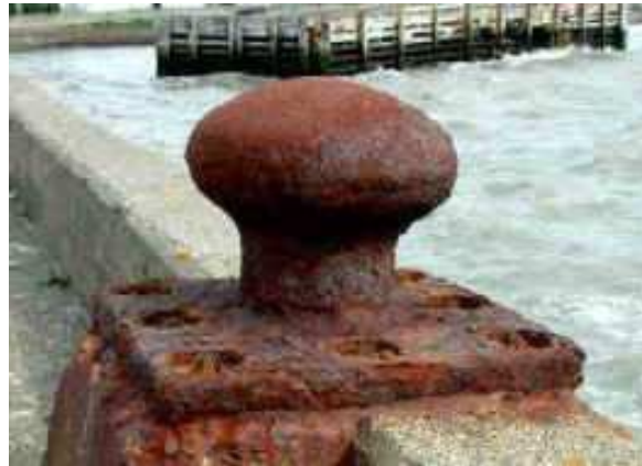
Fig. 2.4 Uniformly corroded steel railing ( Bertolini et al. 2004 )
