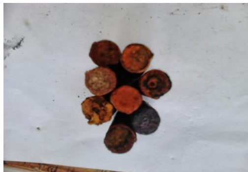
Plate 5.5 – Condition of steel rebars of Type 1 test series at the end of test
