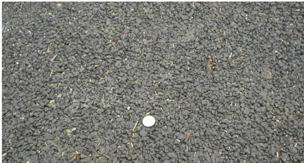
Figure 2. 3 : A Close up View of Porous Bitumen Pavement
