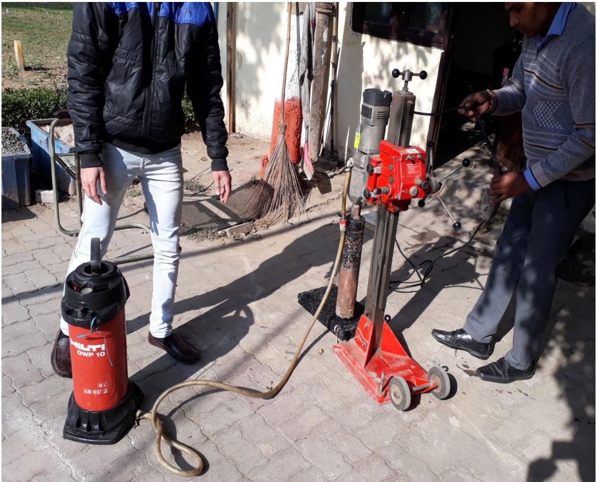
Figure 3. 28 : Core Cutting Machine
