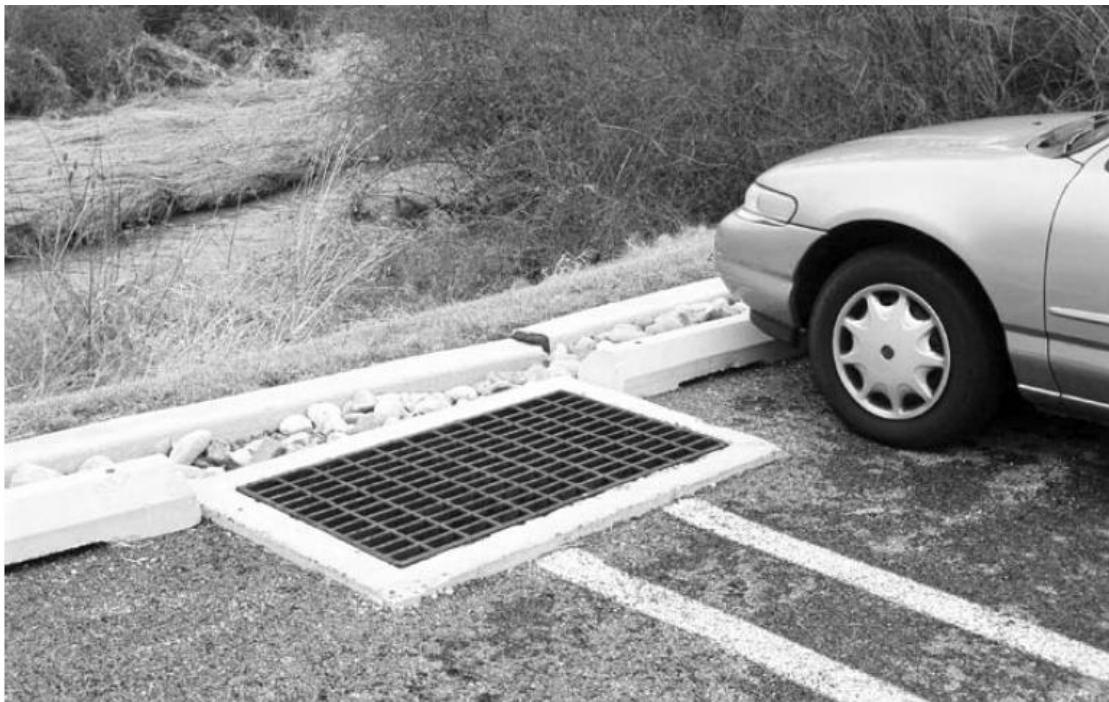
Figure 2. 11 : Permeable Bitumen Parking Area Protecting Stream Water Quality
