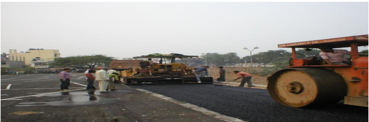
Figure 2. 13 : Typical View of Laying and Compaction of Porous Pavement
