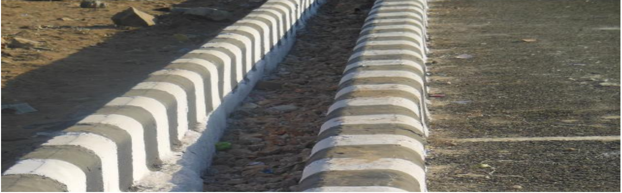
Figure 2. 15 : Close View of Extension of Reservoir Course for Overflow
