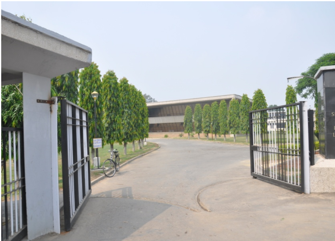
Figure 3.6. Entrance of Research and Development Area
