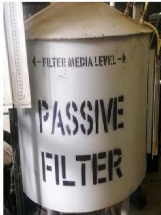
Fig. 3.7: Secondary Filter
