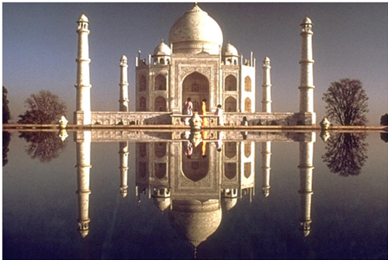
Image enhanced by Riesz approach
