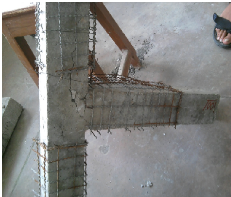
Plate 3.9 Specimen Retrofitted with Mesh Wire
