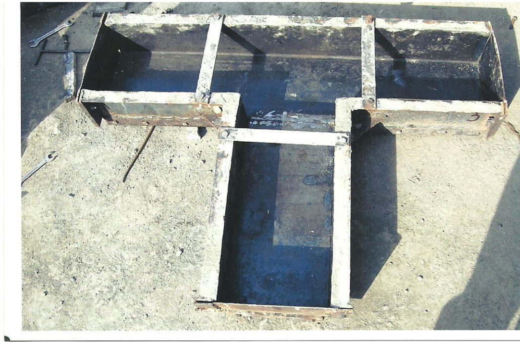
Fig 3.5 Steel Mould for Concrete Casting.
