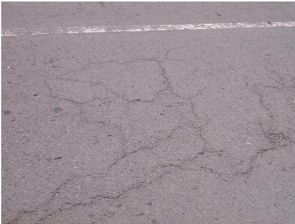
Plate 4.1 Cracked Surface
