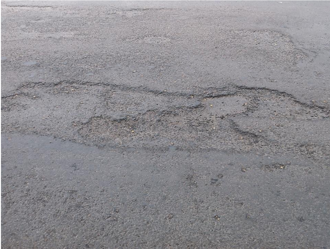
Plate 4.2 Ravelled Surfaces
