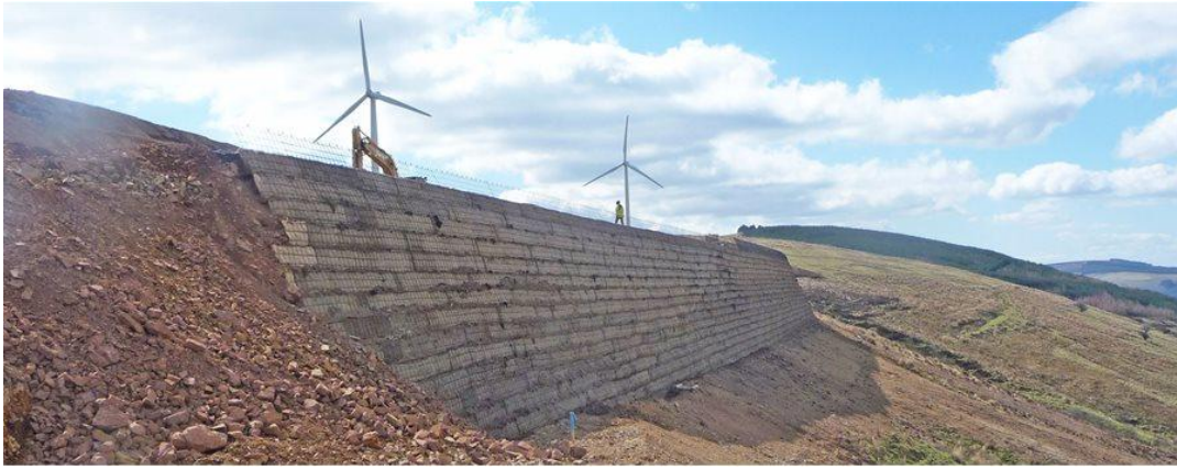
Fig.1.7 (b): Geo-grid in retaining wall construction
