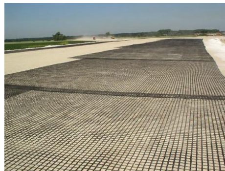
Fig.1.7 (a): Biaxial geo-grid in highway construction
