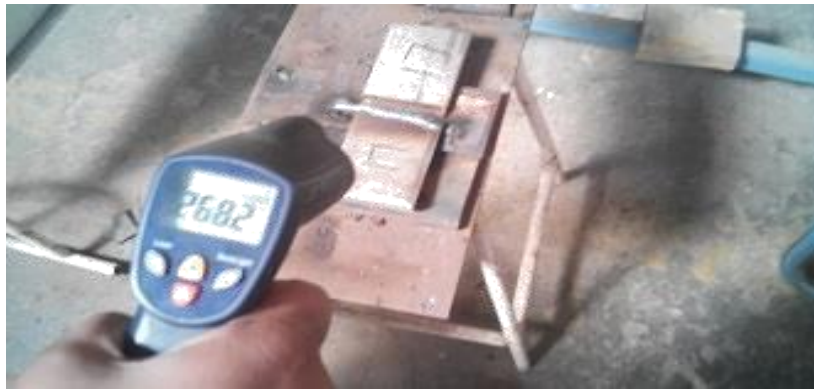
Figure 3.9: Infrared thermometer is used for maintaining interpass temperature.
