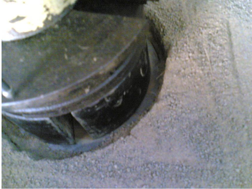
Plate 4.2 Photograph indicating cell, soil, and footing settled together for D=150\text{mm} ( d/D=1.0 )
