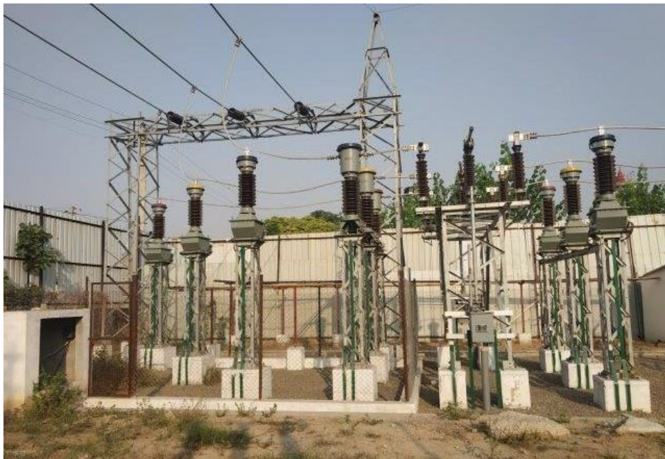
FIG.1.2: CT/PT MOUNTING ARRANGEMENT
