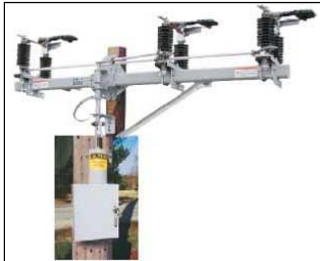
Figure 2.1 Pole Top RTU [19]
