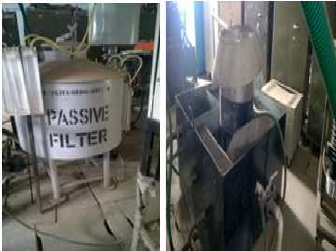
Figure 5.9: Passive filter and cooling unit
