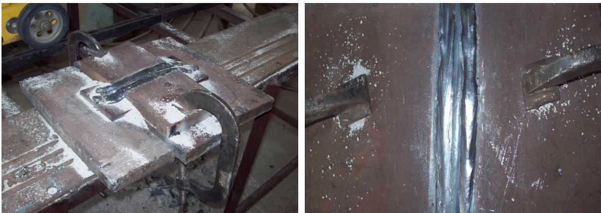
FIGURE 3.13- Joint of plates after welding
