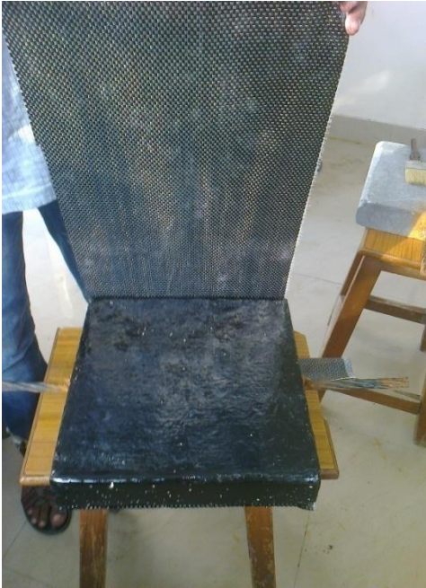
Fig.6.10 Placing CFRP sheet
