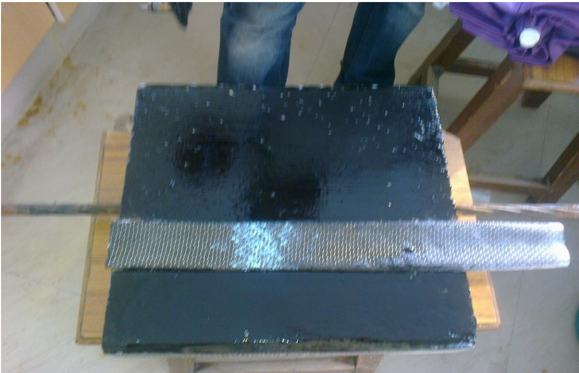
Fig.6.9 Epoxy applied on concrete surface of slab
