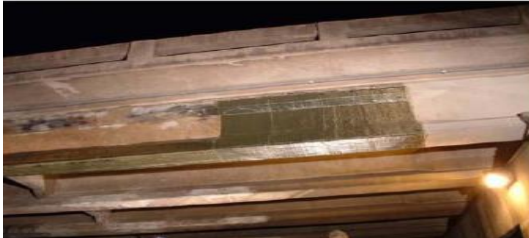
Fig. 4.2 FRP Wrapped around Corroded part in Bridge
