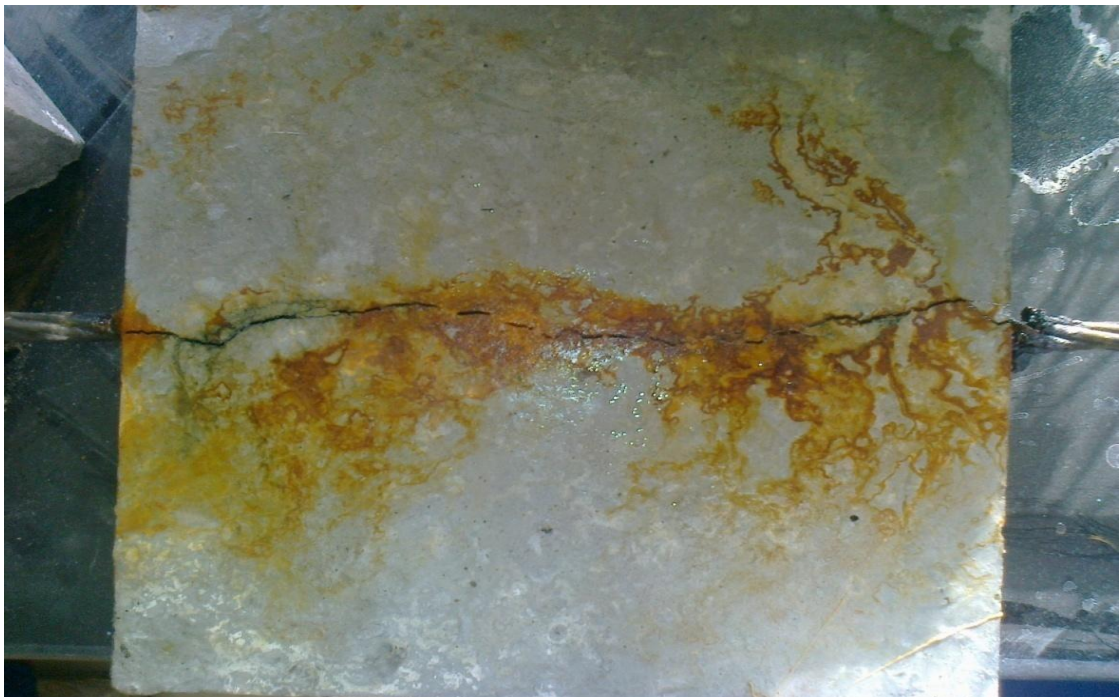
Fig. 7.5 Longitudinal crack along the length of Strand
