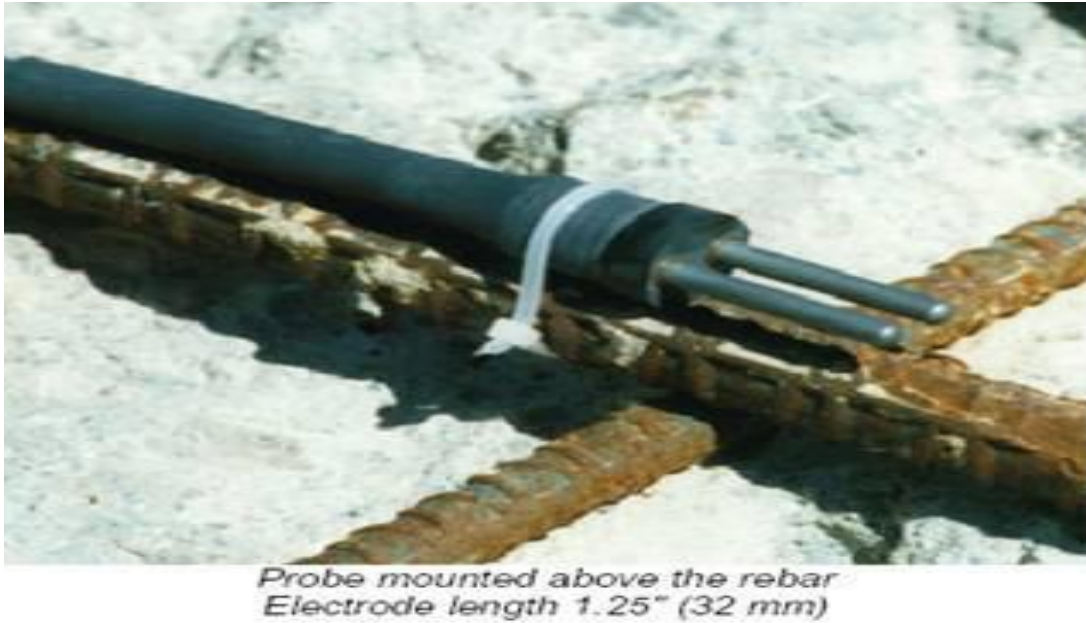
Fig. 2.10 A LPR probe installed in a concrete structure.
