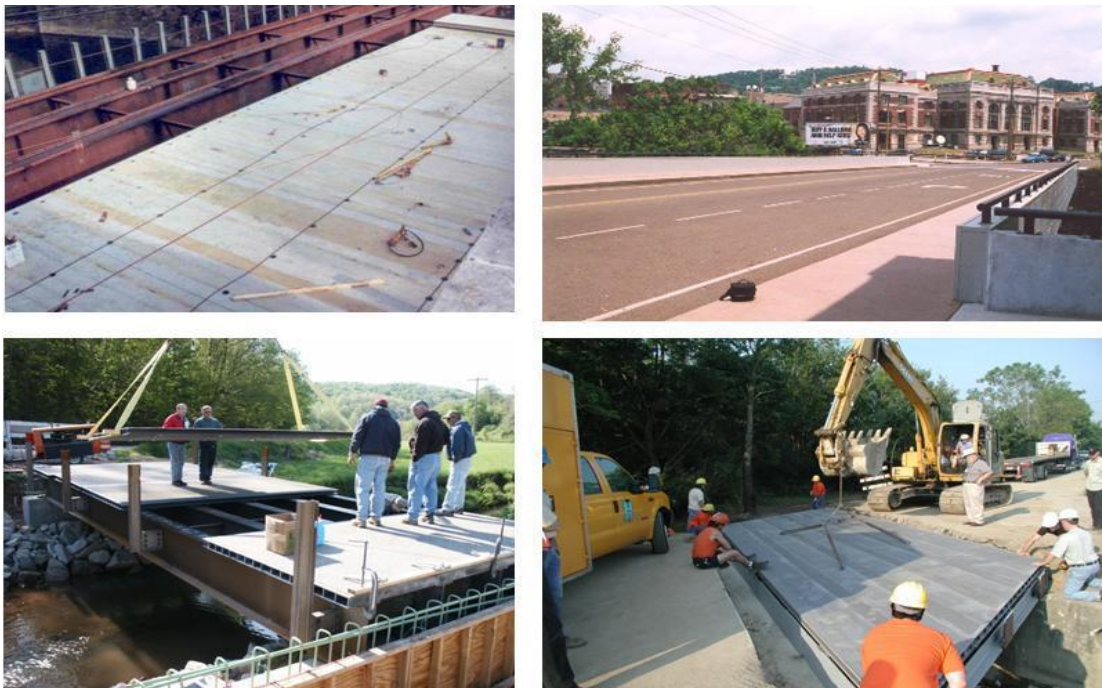
Fig 4.7 FRP bridge deck shapes designed and field implemented in WV and Ohio by the CFC-WVU (Courtesy: CFC-WVU)
