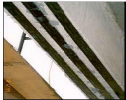
Flexural Strengthening
