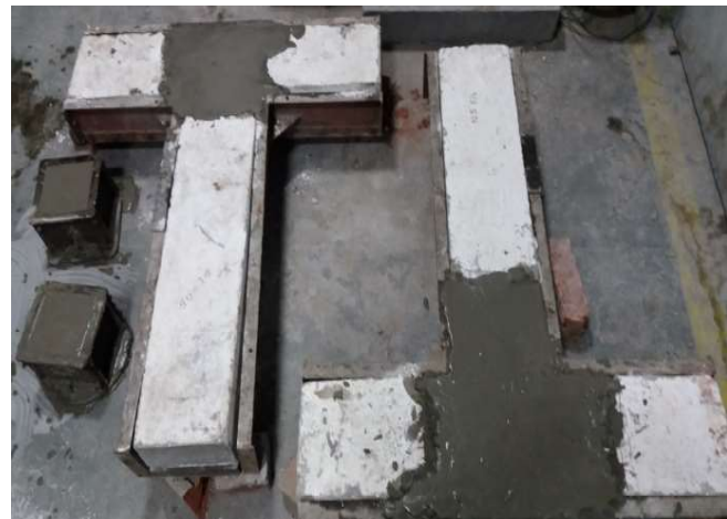
Figure 3.12 (c): Retrofitting done.
