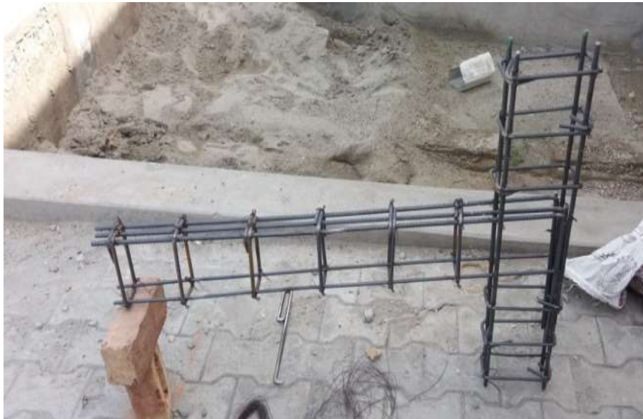
Figure 3.9 (a): Formation of steel mesh
