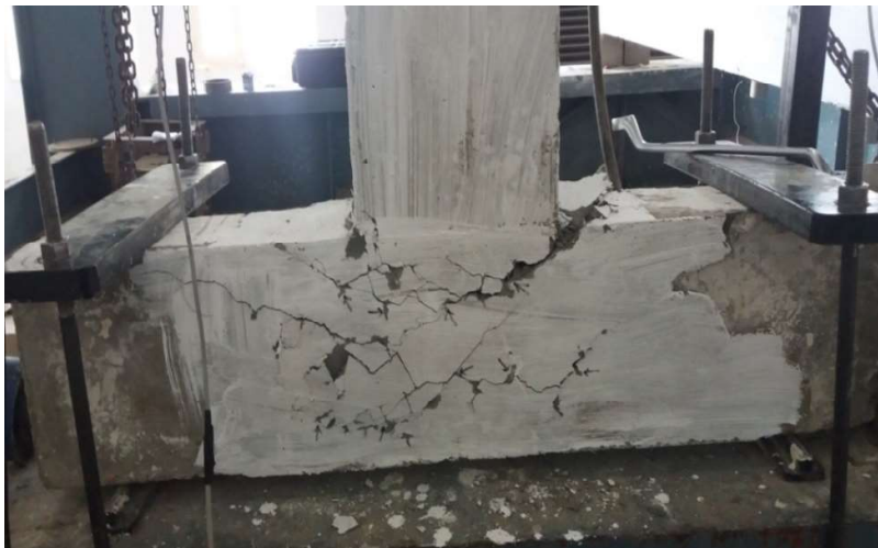
Figure 4.1 (b): Cracks formation after retrofitting.
