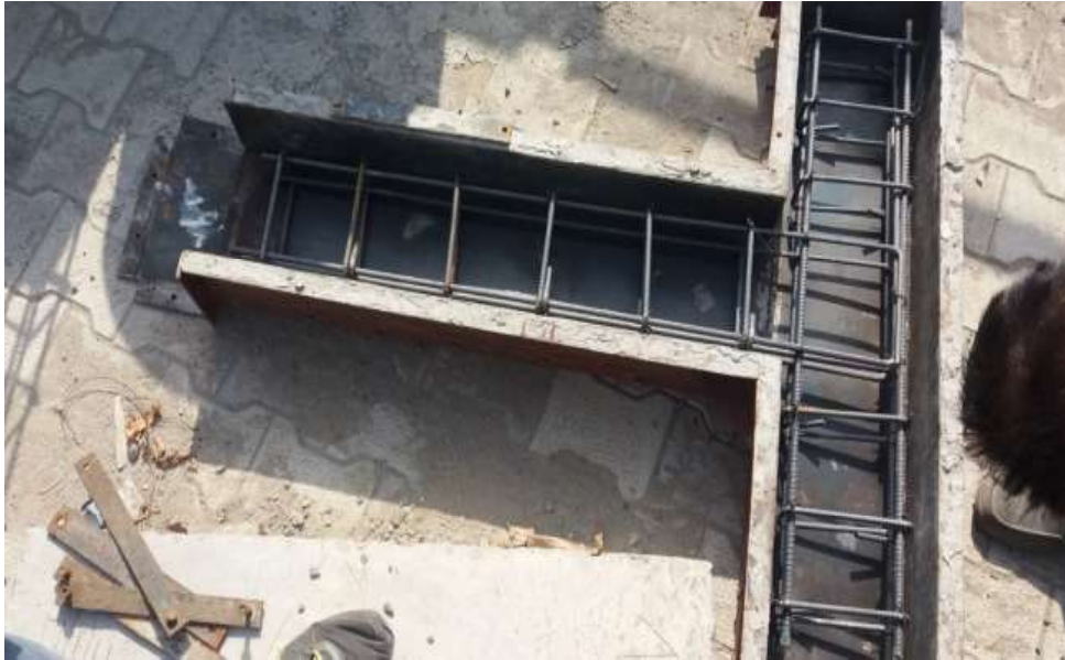
Figure 3.9 (b): Placement in mould.
