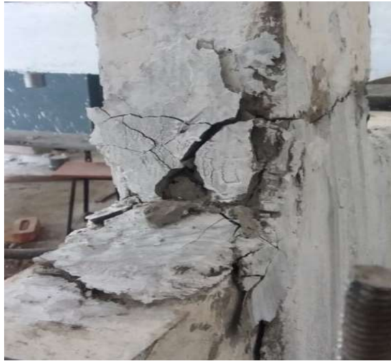
Figure 4.7 (d): Fibres preventing spalling of concrete specimen S2..
