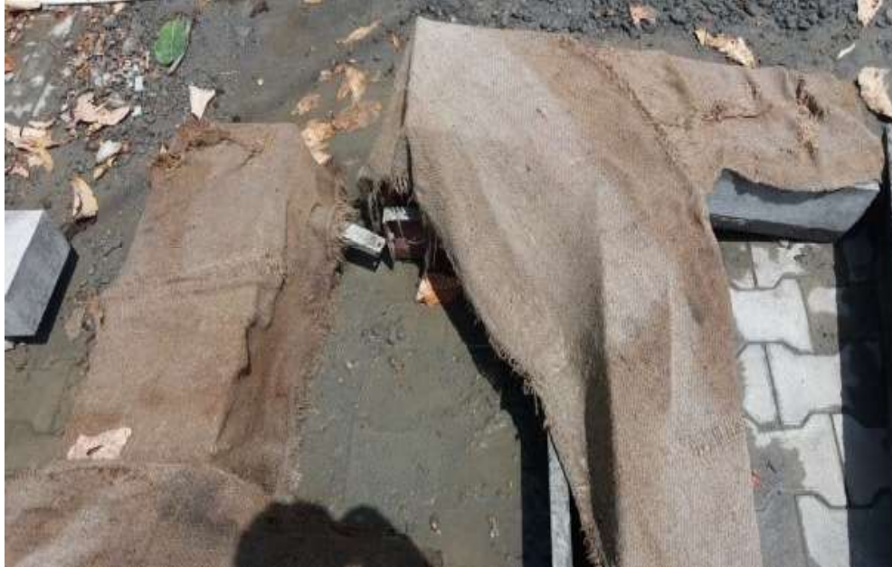
Figure 3.9 (d): Curing of specimen.
