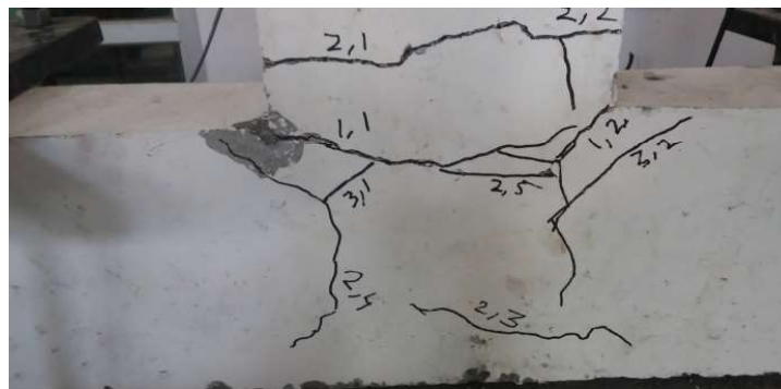
Figure 4.7 (a): Cracks formation prior retrofitting for specimen S2.
