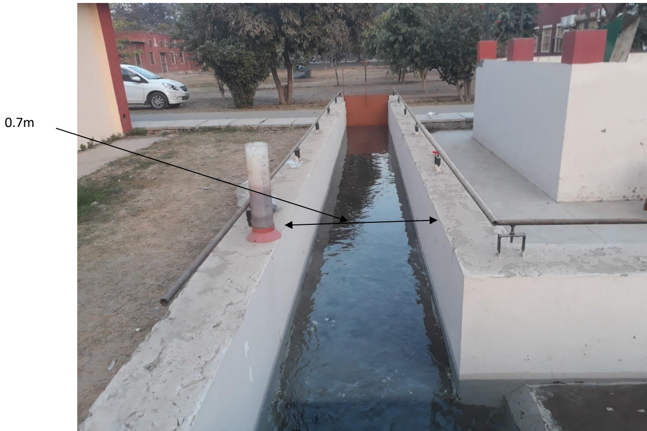
Figure 3.4 Open channel with instrument fastener
