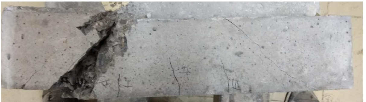
Figure 4.34 Cracks in G3 (2) of grade M35 beam at ultimate load 56.93kN
