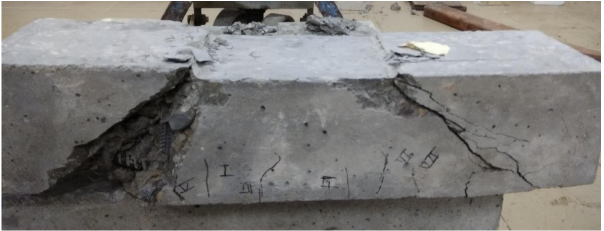
Figure 4.37 Cracks in G4 (1) of grade M35 beam at ultimate load 73.86kN
