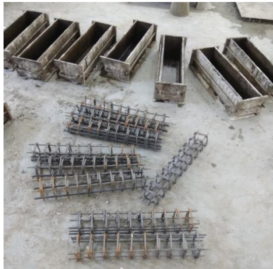
Figure 3.10 Oiled moulds with Steel and GFRP arrangements of beams
