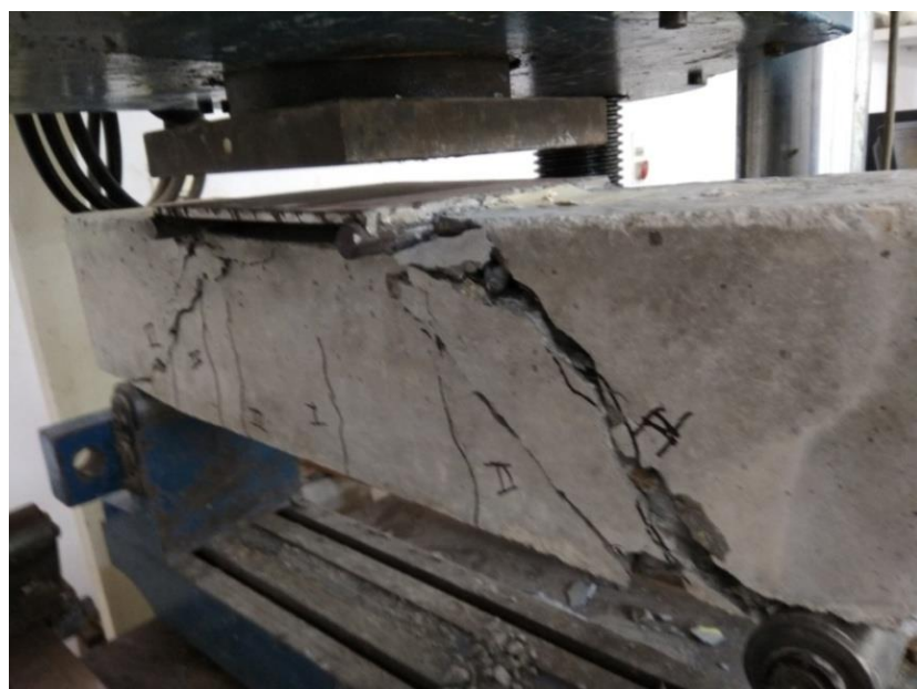
Figure 4.24 Cracks in G1 (2) of grade M30 beam at ultimate load 52.7kN
