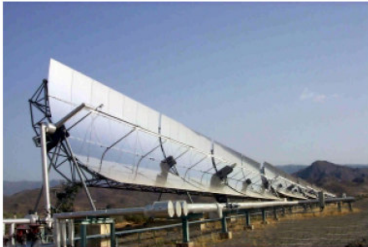
F 4.8 - Showing medium concentration solar collectors.
