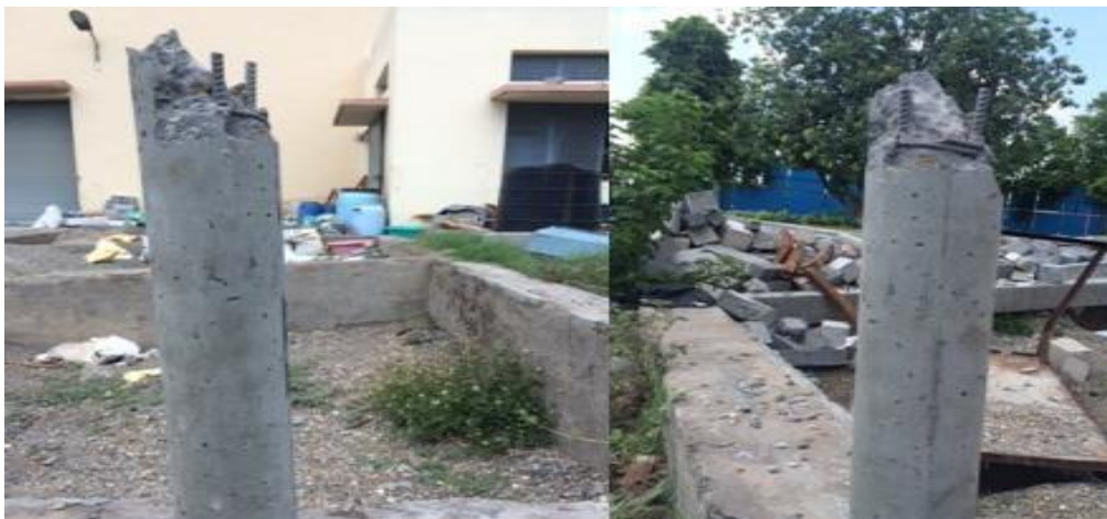
Fig. 4.9 Detail of column during final phases of loading
