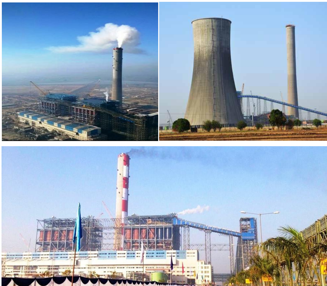
Figure 4.6 General view of the Rajpura Thermal Power Plant
