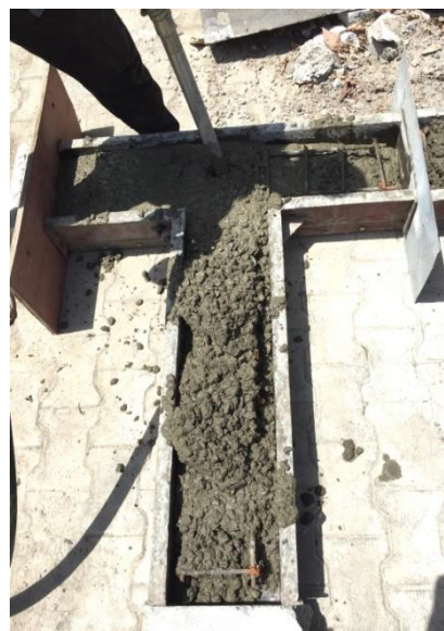
b) Compaction of Concrete using Vibrating Needle
