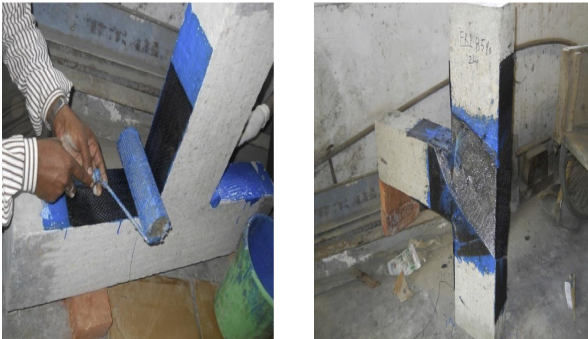
Figure 2. 6 Retrofitting with CFRP (Singh.V et al. 2014)
