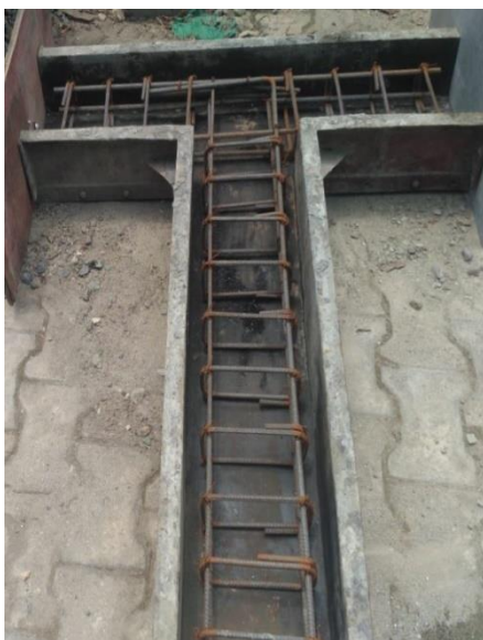
a) Reinforcement Cage in Moulds
