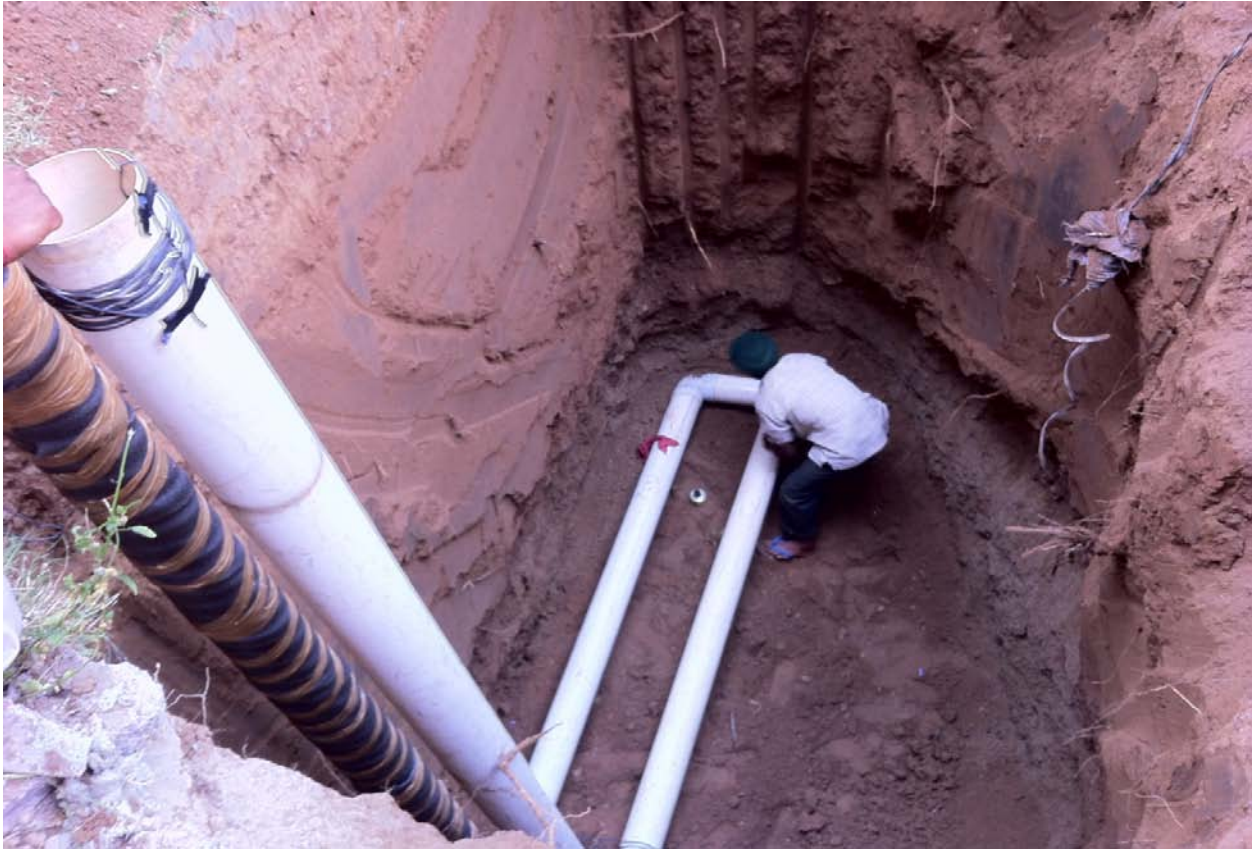
Figure 5.4: Experimental Set-Up after installation in trench.
