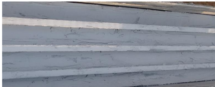
Fig.3.5 Adhesive Bonding on GFRP Plank
