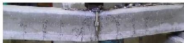
3) Flexural failure of specimen C2
