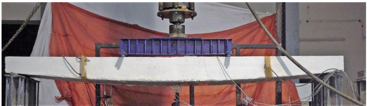
Fig.4.45 Hairline Cracks on the Surface of CG Slab after 3 rd Cycle
