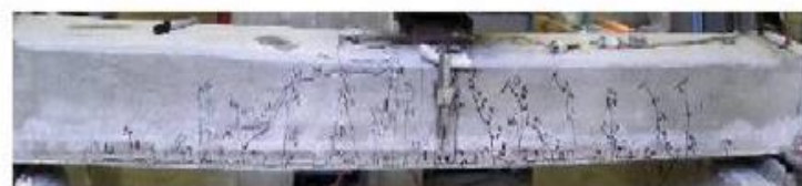
2) Hybrid failure mode of specimen 5
