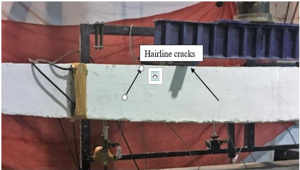
Fig.4.54 (a) Hairline Cracks Appeared on the Surface of CA Slab at the End of 2 nd Cycle
