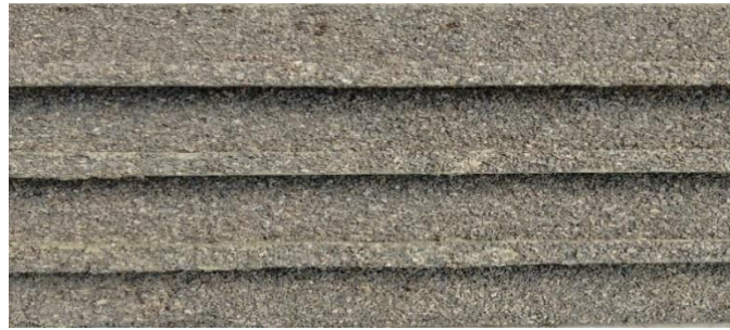
Fig.3.4 Aggregate Bonding on GFRP Plank
