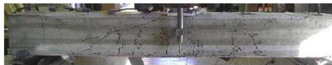
a) Shear failure of specimen 1
