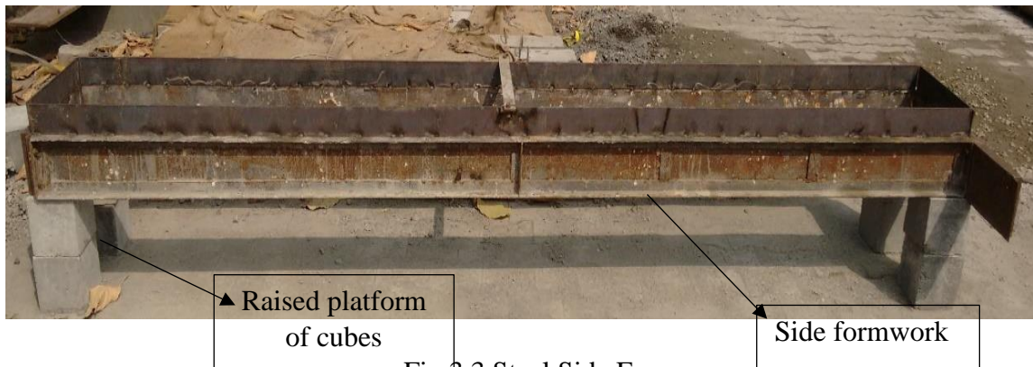
Fig.3.3 Steel Side Form
