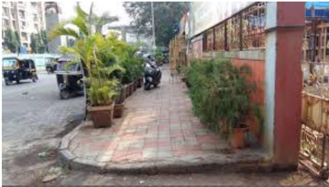
Figure7.1: Encroachment of Sidewalk by House Owner and Parking of vehicle on sidewalk leaves little space for adequate pedestrian usage.
