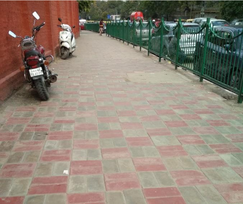
Figure5.1: Sidewalk, Laxman Public School, Hauz Khas
