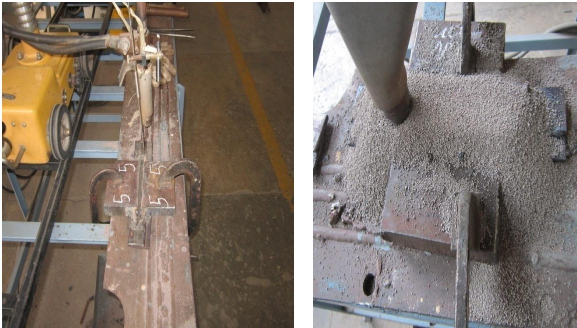
FIGURE 3.13 Submerged arc welding of plates after single layer
