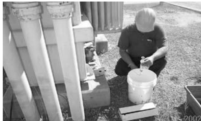
Figure 3.1 Working process of Dissolved Gas Analysis (DGA)
