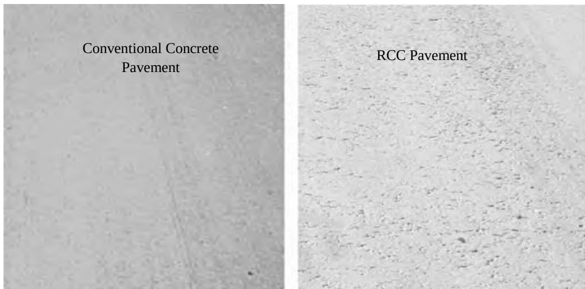
Fig. 1.3: Surface texture of conventional concrete pavement and RCC pavement ( Harrington et al., 2010 )
