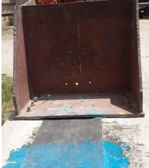
Fig 3.10 Pasting of Sheet and Fixing of Prestressing Machine
