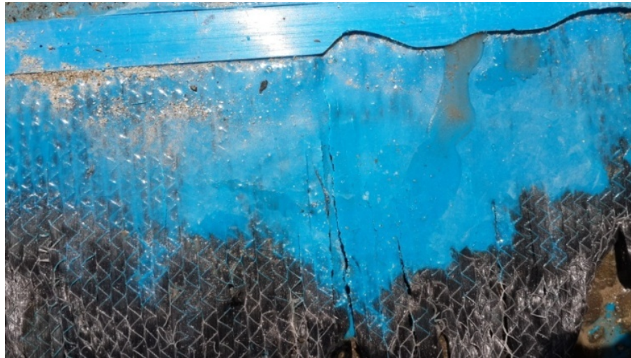
Fig. 4.1 Tensile Cracks in S1 Sample
