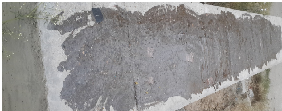
Fig. 3.9 Beam Primed with Master Brace 3500 Primer
