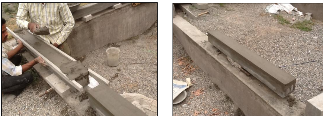
Fig. 3.4 Columns Confined with Mortar Layer
