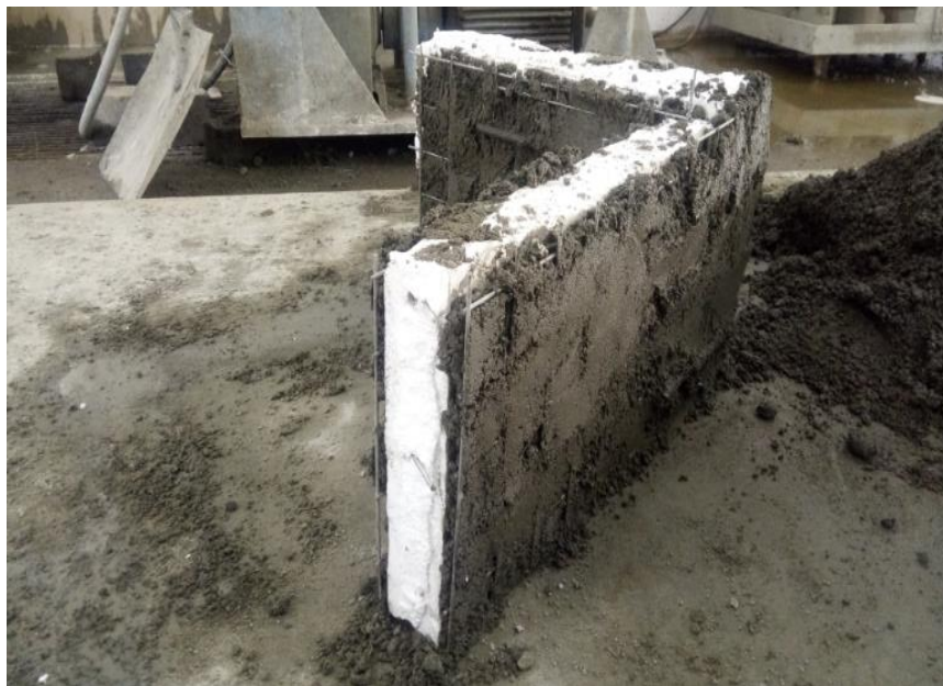
Figure 3.14 L-shaped connection after applying the first layer of mortar
