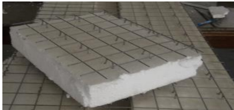
Figure 3.12 Cutting of EPS panels
