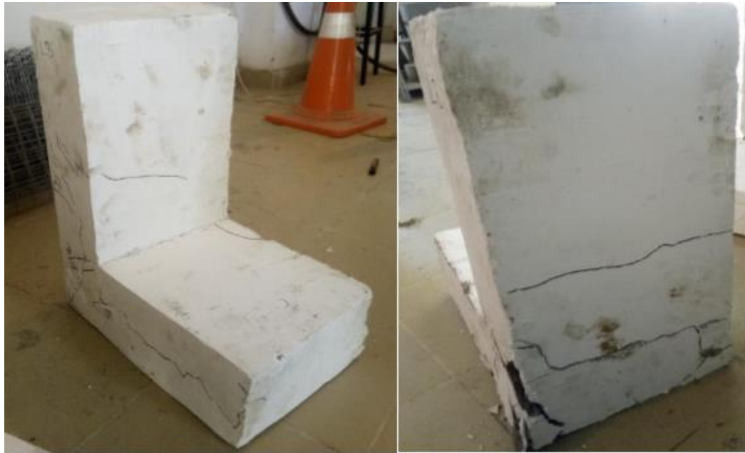
Figure 4.4 Cracks developed in L3 during testing
