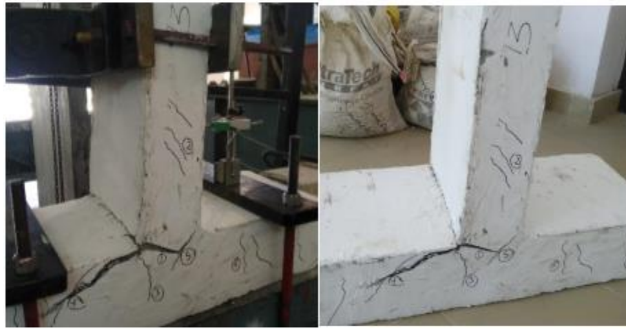
Figure 4.9 Cracks developed in T3 during testing
