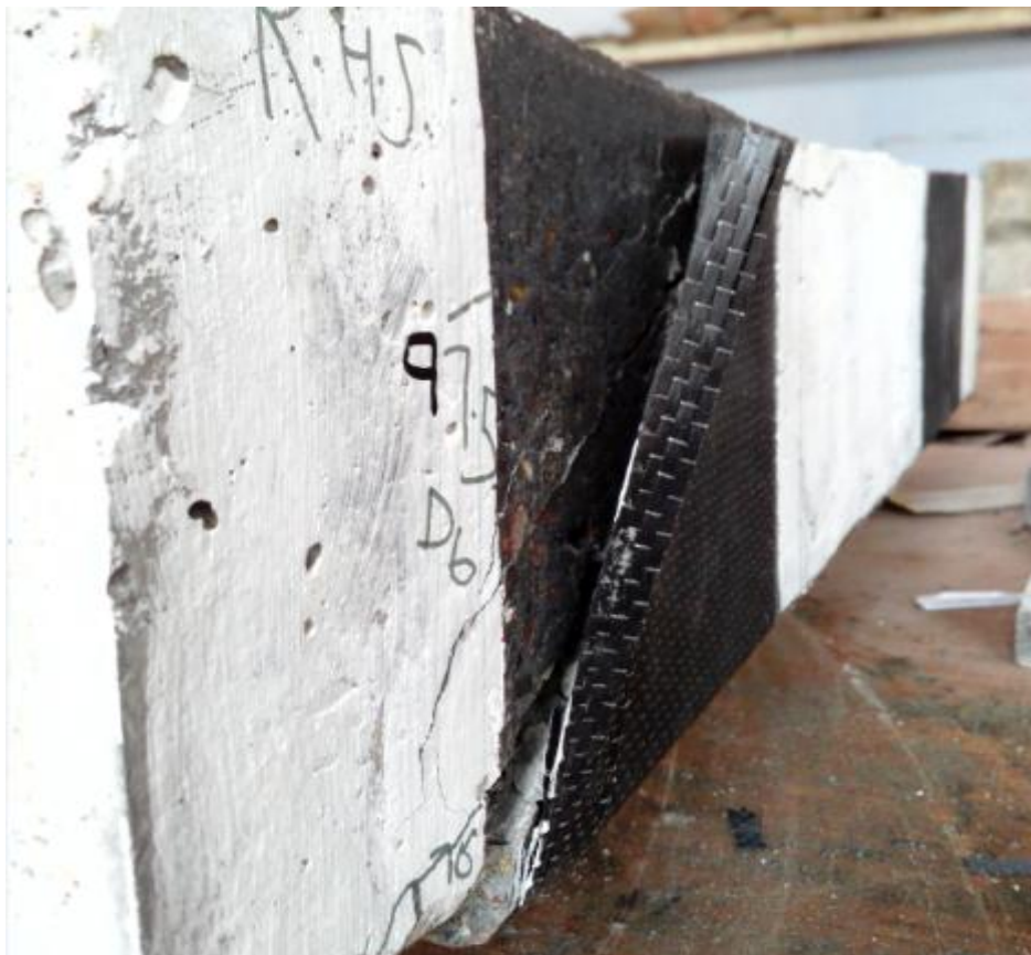
Figure 4.15 – Debonding of CFRP U-wrap in strengthened beam SB-05
