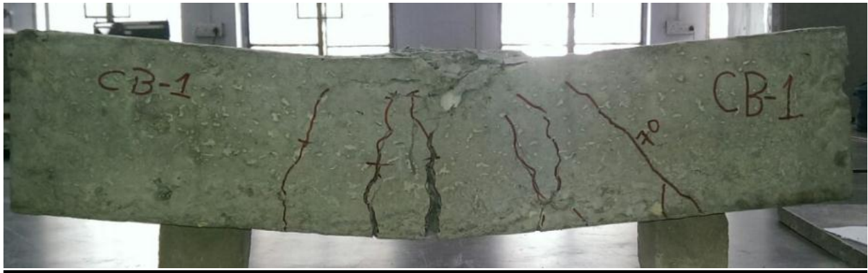
Figure 4.2 – Crack patterns in control beam CB-01at failure
