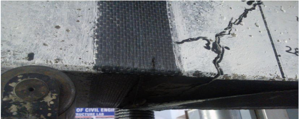
Figure 4.32 –Plate End Debonding in strengthened beam SB-13
