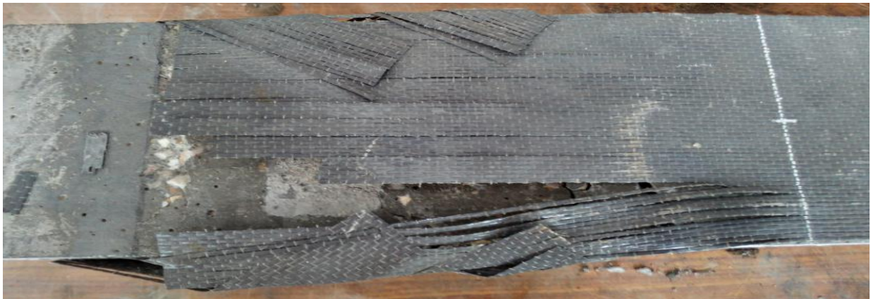
Figure 4.21 – Plate End Debonding in strengthened beam SB-08
