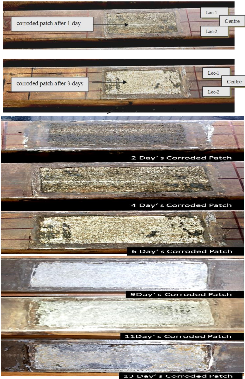
(b) Corroded patch after exposure of increasing days of corrosion
