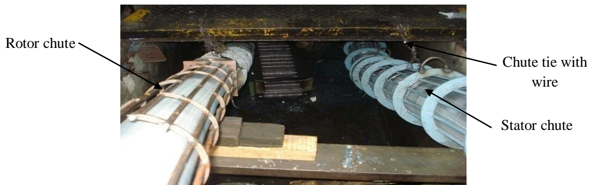
Figure 4.6: Old process of clamping the free end of chute [Crompton Greaves, Ahmednagar]
