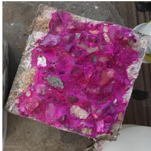
Fig. 3.23: Change in colour of concrete after application of phenolphthalein solution on split cube sample
