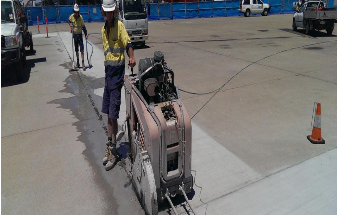
Fig. 1.4: Saw cut in transverse direction
