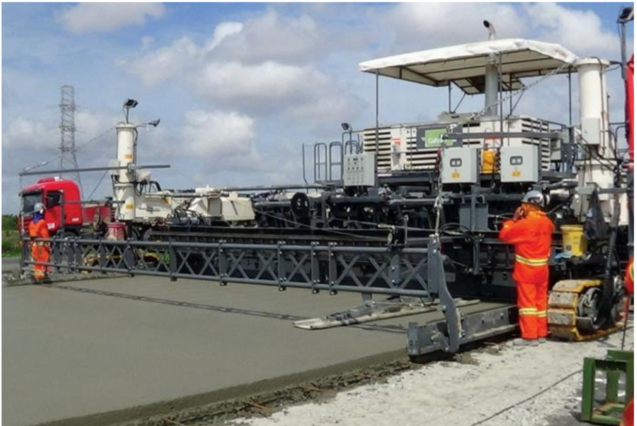
Fig. 1.8 Laying of Pavement Quality Concrete (PQC)
