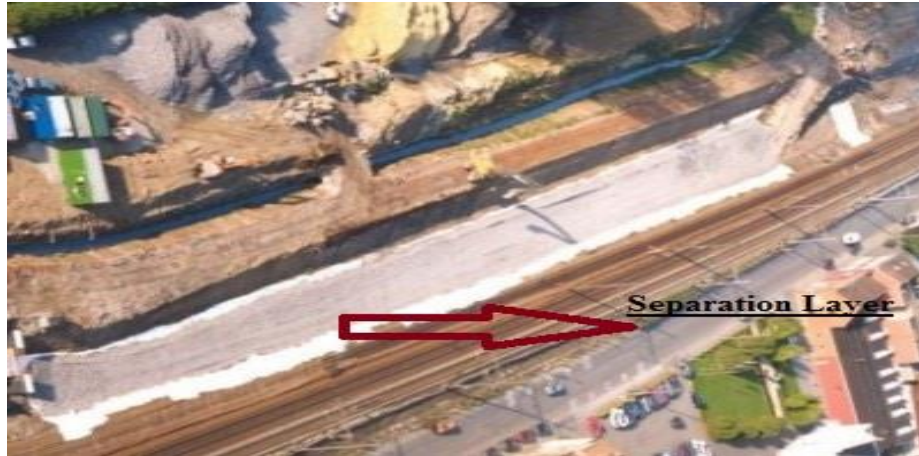
Fig. 1.2: Laying of separation membrane
