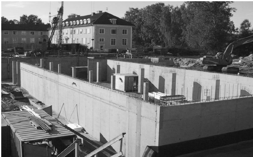
Figure 1.9: RCA use in New High School construction in Sorumsand, Oslo, Norway, ( www.irbnet.de )
