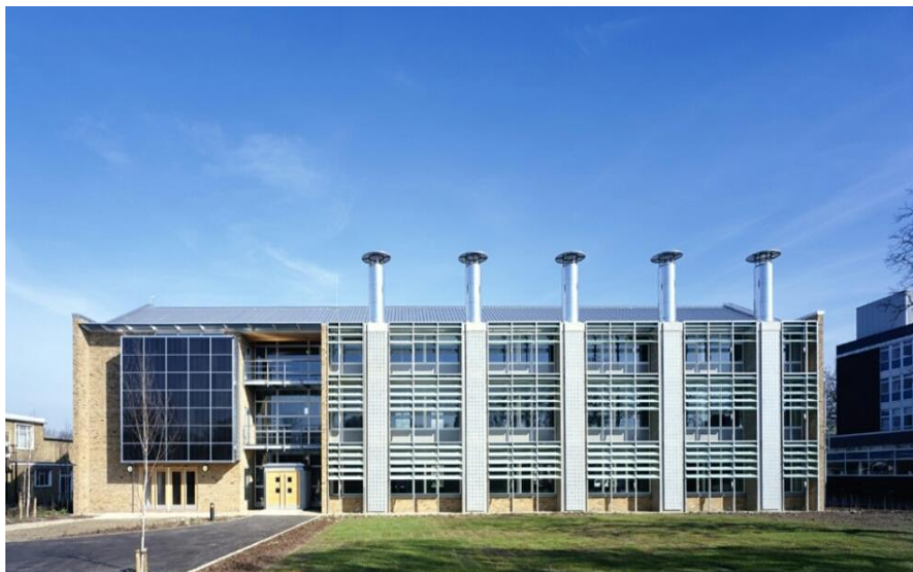
Figure 1.7: Shows the front view of the BRE office Building, Garston, Watford, UK, ( https://fcstudios.com/work/view/new-environmental-office-bre )
