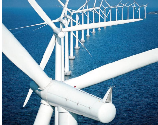
Figure 1.3 Applications of optical fiber sensors: turbine blades.
