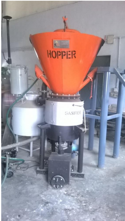
Fig 28 Down draft gasifier setup
