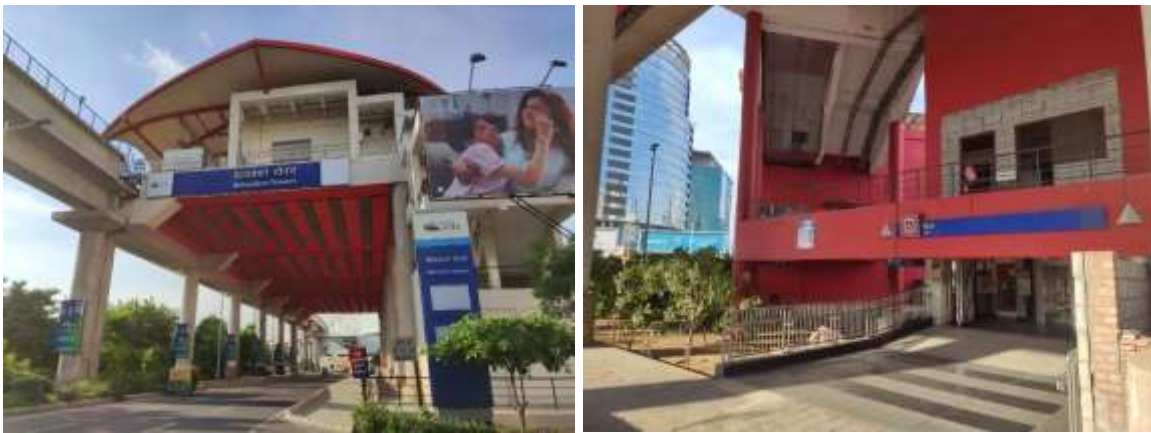
Fig: 4.19 Pedestrian access facilities at Belvedere Towers
