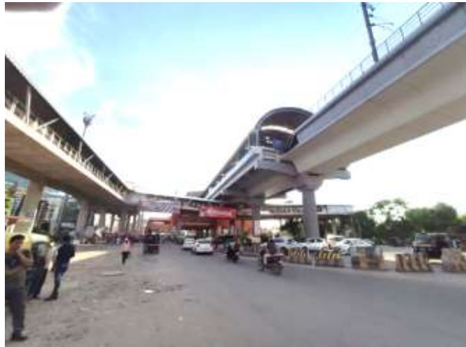
Fig: 4.21 Foot over bridge on Sikanderpur Metro Station
