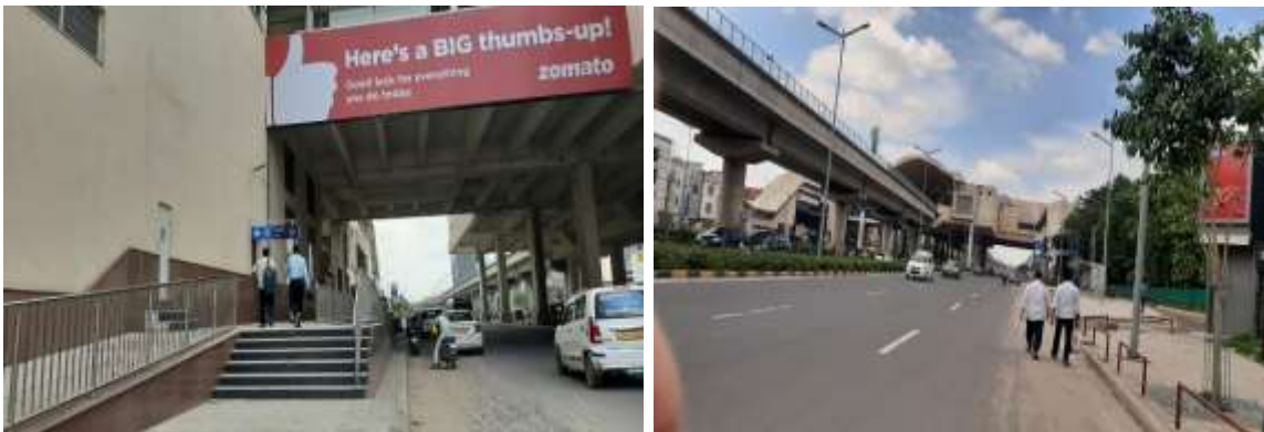
Fig: 4.20 Ramps & side walk with guard rails at Sector-43 Station
