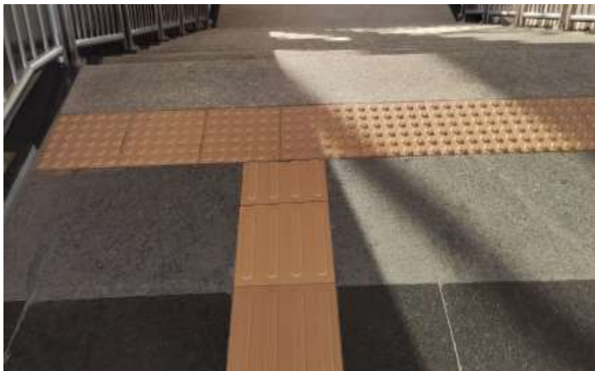
Fig: 4.22 Adequate floor pattern or braille signage for blind people at metro station
