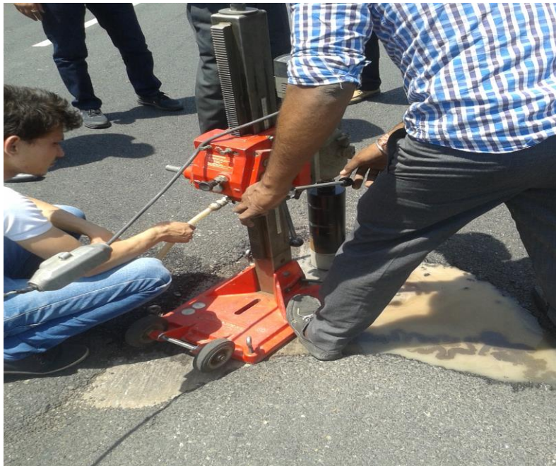
Plate3.9: View of Instrument of Test Pit Testing
