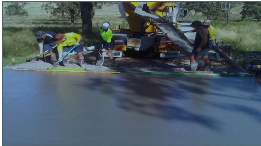
Fig 1.4: Placing of Pavement Using Geopolymer Concrete ( Aldred and Day 2012 )
