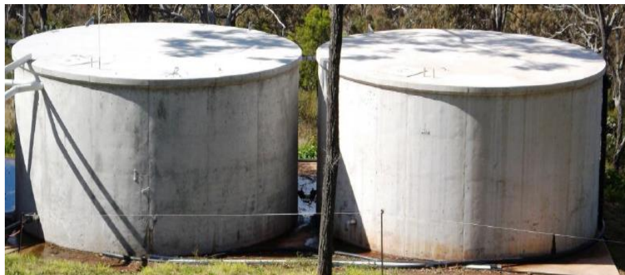
Fig 1.5: In Situ Water Tanks, Cast with Geopolymer Concrete (Right) and Cast with Cement Concrete (Left) ( Aldred and Day 2012 )
