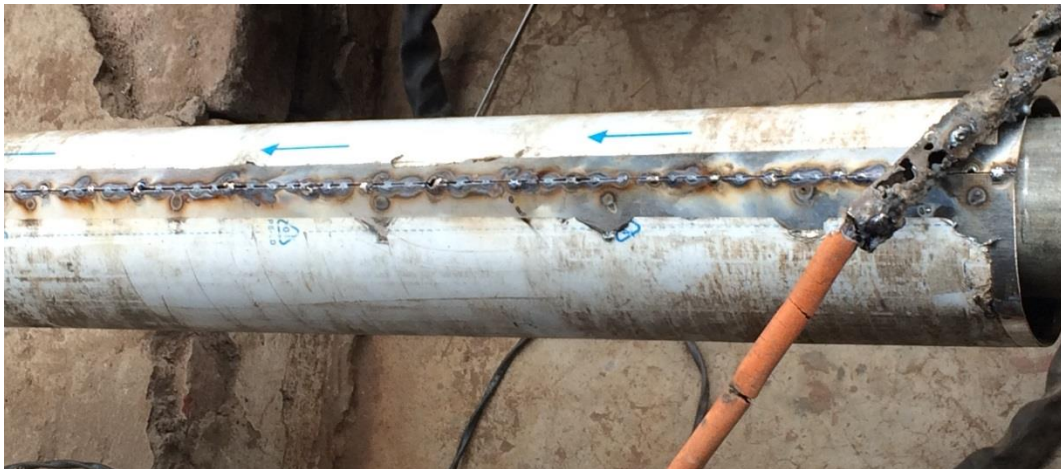
Fig. 4.16 welding of cylindrical sheets
