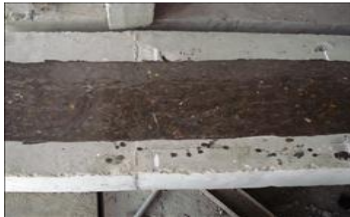
Fig 3.6 Surface after Grinding and Priming
