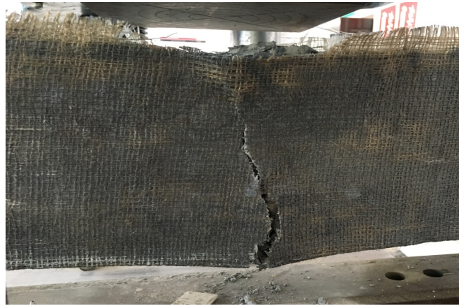
Figure 4. 15 : Clear view of crack showing flexure failure of UW-B1 beam at failure.
