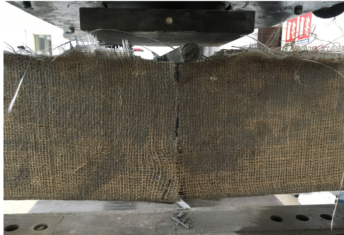
Figure 4. 20 : Showing crack pattern of UW-B3 at ultimate failure load.
