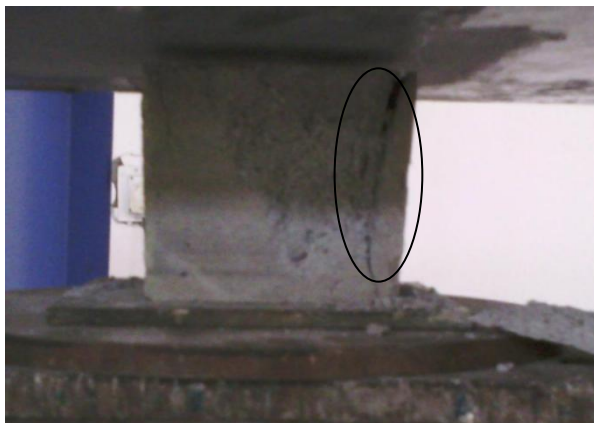
(c) Actual Image at failure
