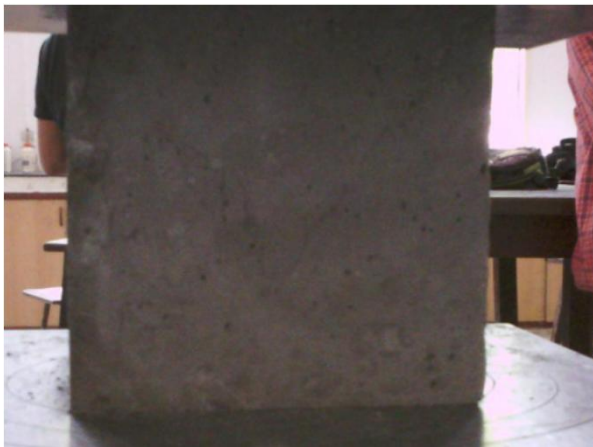
(c) Actual image at first major crack
