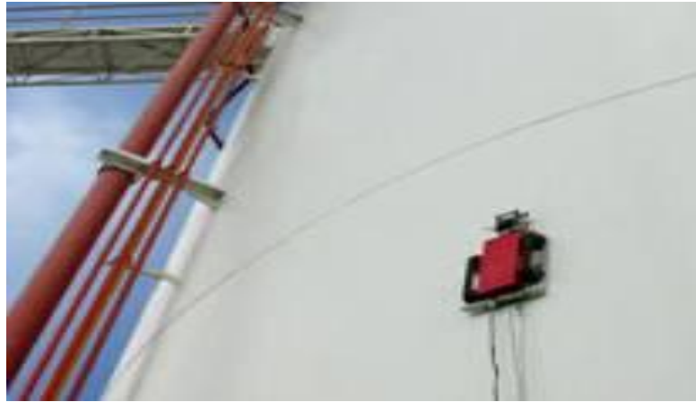
Figure 1.1 Storage tank inspection [1]
