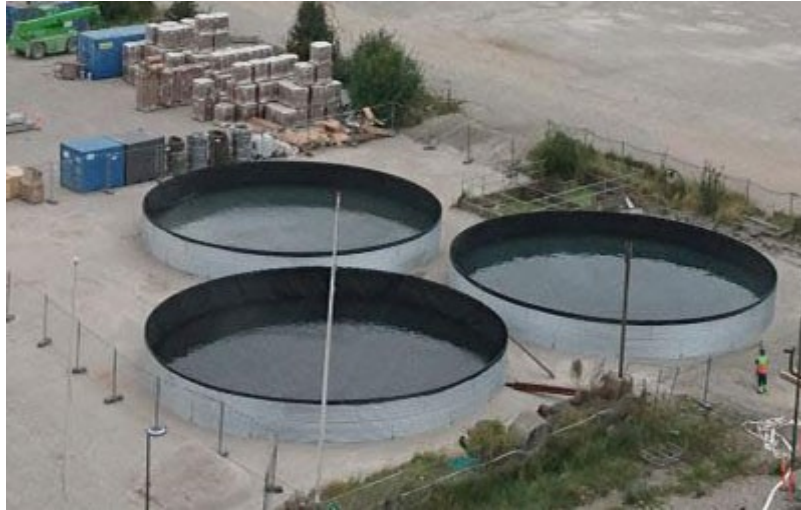
Figure – 5.9 Tanks for storage of Water ( https://www.butylproducts.co.uk/2016/08/25/steel-water-storage-tanks/ )
