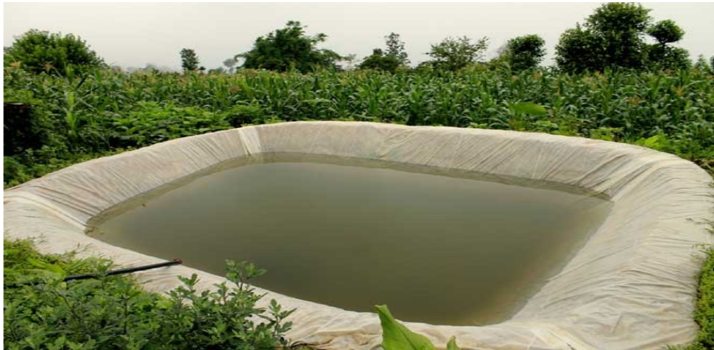
Figure 5.8 Water Storage Pond
